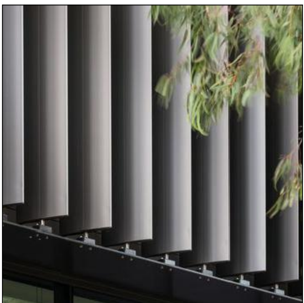
PS2 PRIVACY SCREEN VERTICAL BLADE SCREEN TO MATCH AFG FINISH OR SIMILAR
